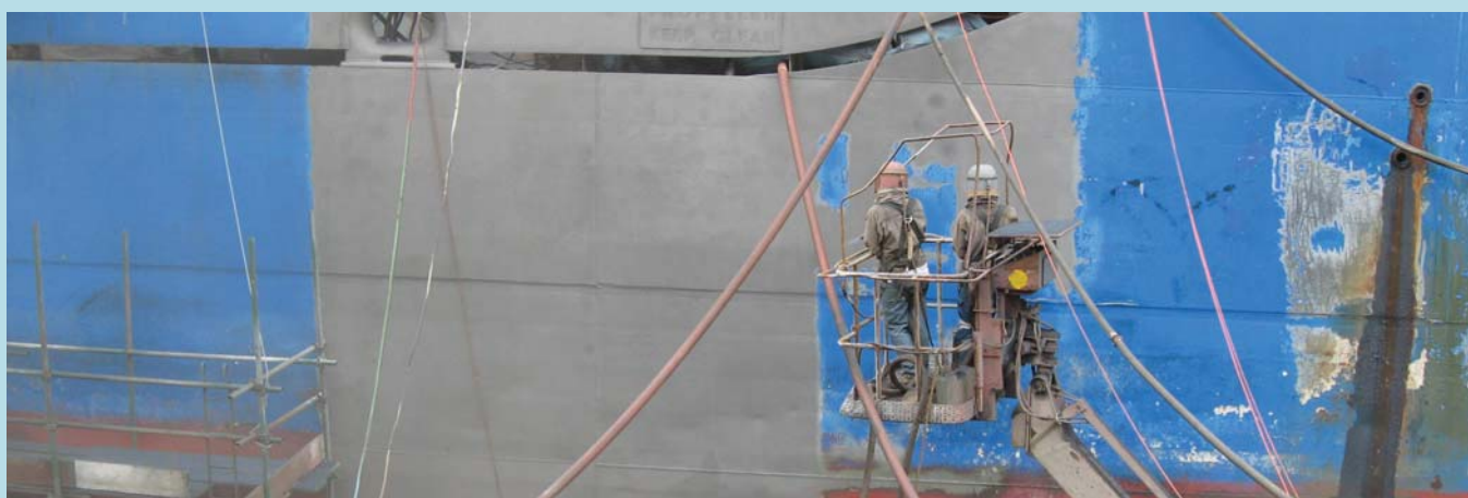
Repainting the JOIDES Resolution hull in dry dock.
