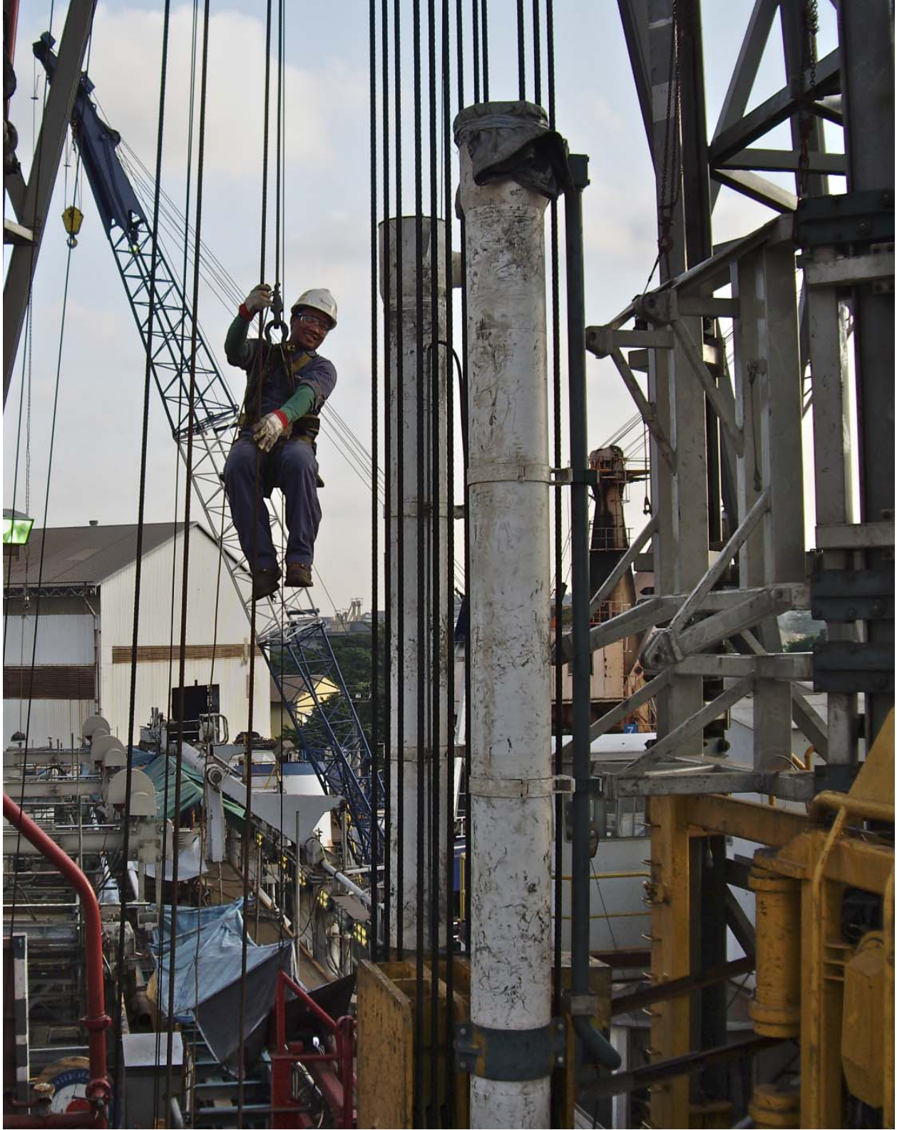
Installing the refurbished passive heave compensator.
